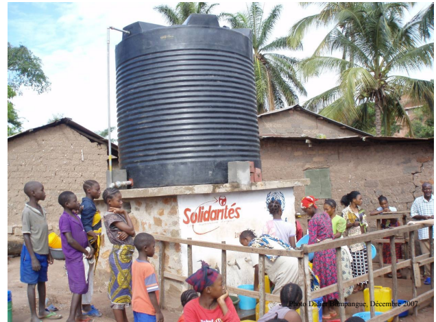
Figure 5. Waterpoint system implemented in Kalemie by NGO Solidarités.
