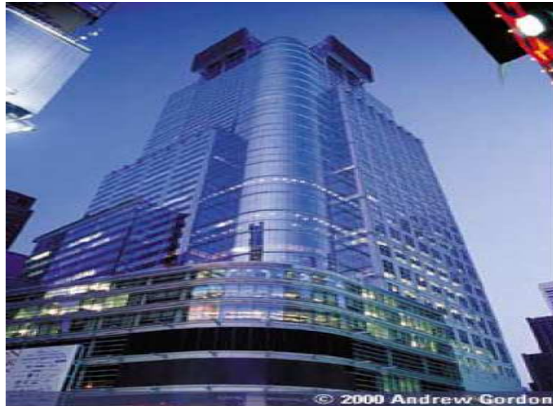
Fig. 1.10. Building in New York's Time Square (photo courtesy of Fuel Cell 2000).
